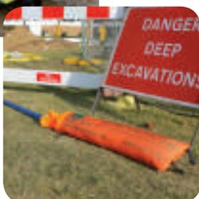
UK Power Networks are trialling new polymer-membrane technology as an alternative to conventional concrete bunds at two locations
